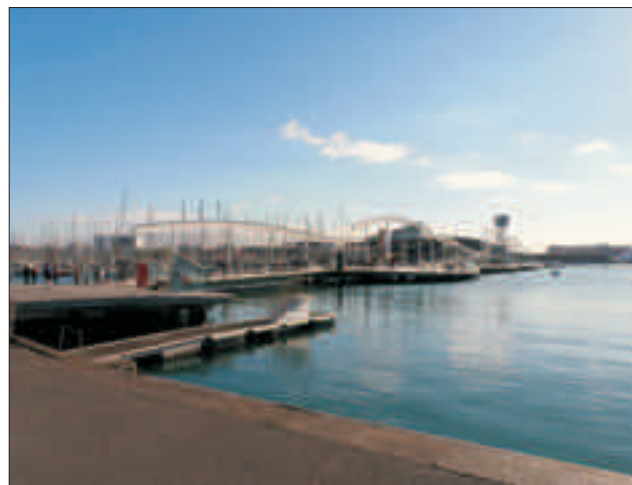
Figure 6.31. Connection of the historic city to the harbour area (photo N. De Maesschalck).
