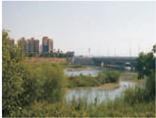
Figure 2.18. Boğaçay Stream and the bridge over it on Akdeniz Boulevard.
