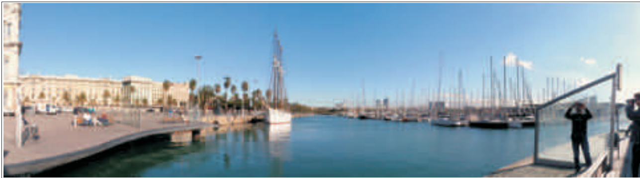
Figure 6.29. Moll de la Fusta after reconstruction (photo N. De Maesschalck).
